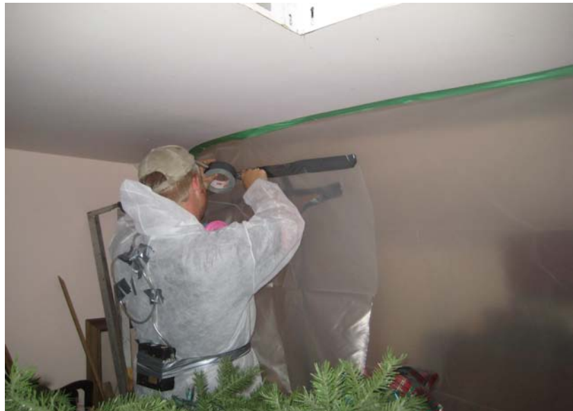
Figure A14: Crew member building containment prior to wall blow-in.
