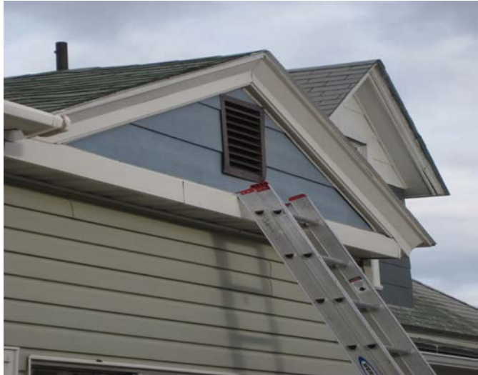
Figure A6 Exterior attic access installed by weatherization crew member.
