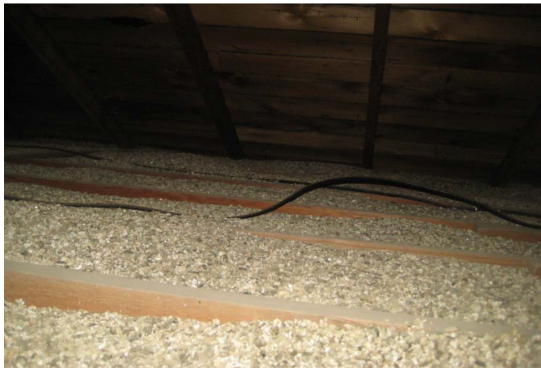
Figure 1 Example of asbestos-containing vermiculite attic insulation.
